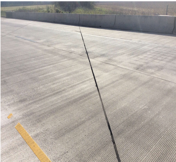
PHOTO 1 Description Bent #2,3 pourable joint has a few feet each bent with loss of adhesion 20 feet total.
